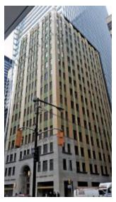
The south and east elevations of the EY Tower in Toronto are comprised of a mix of Roman Stone, terra cotta and new heritage-style bricks up to the 14th storey. - Photo: CLIFFORD RESTORATION
