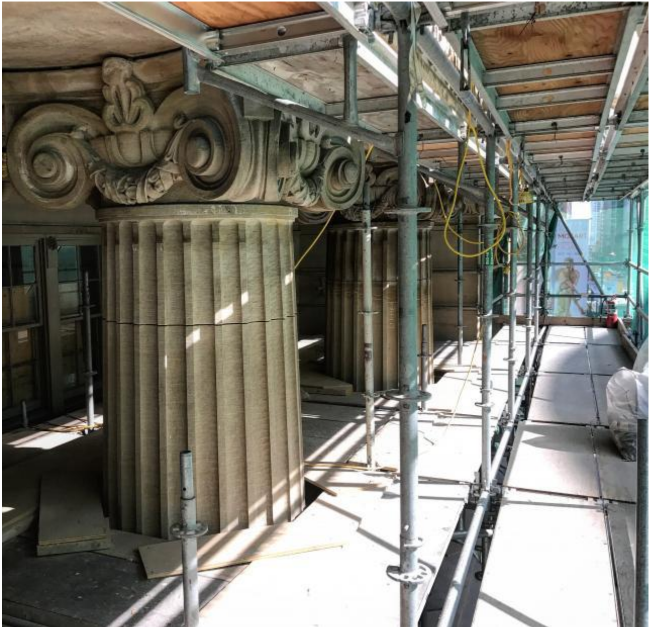
Stonework being restored at the Massey Tower, image by Gary Switzer
